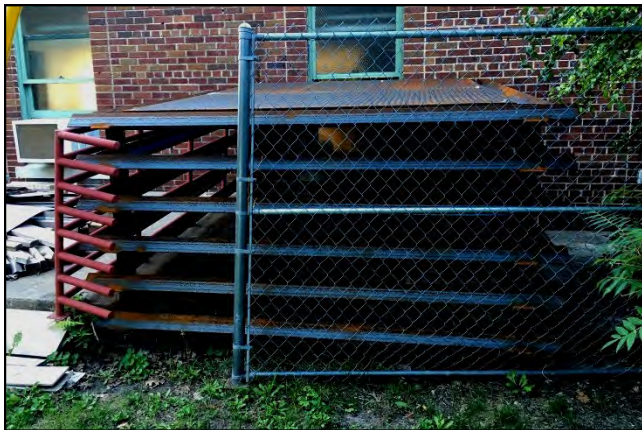
A cupola-style bat-friendly gate was constructed over the entrance to an underground walkway at Lake View Hill Park in Madison in an effort to make the site accessible to bats for hibernation.
