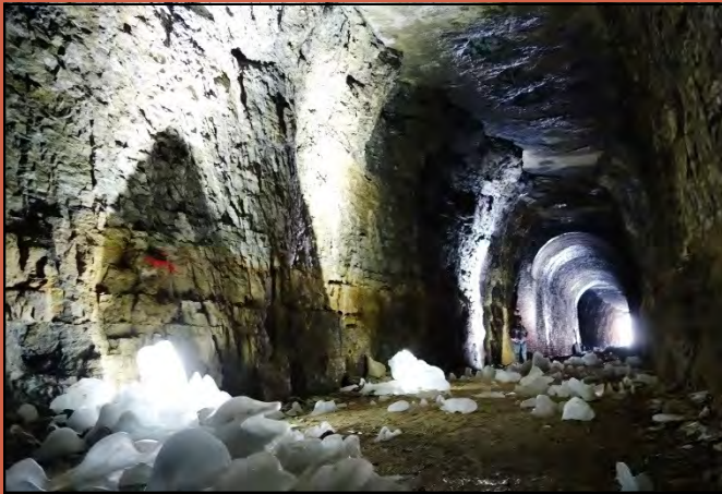
Unusual ice formations build up as water drips from a state trail tunnel ceiling, indicating the freezing temperature created as air is drawn through the open ends of the tunnel in winter.
